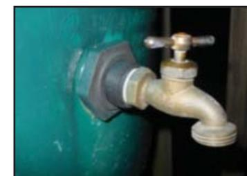
Spigot attached to a bulkhead tank fitting
